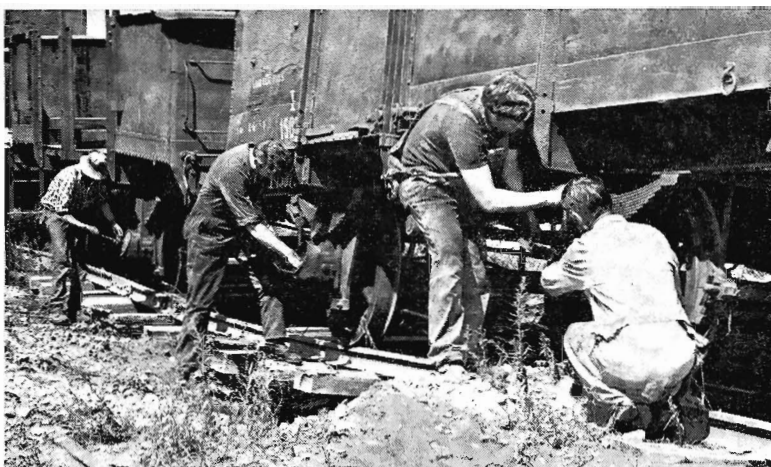
After the flood, every wagon in Orbost yard—more than 100—had to have its brake gear and axle boxes examined and cleaned of silt. Going about their monotonous task in a flood damaged road when News Letter visited the area, were (from right to left) Traralgon Depot Foreman D. Robson, Train Examiner D. Westland, Fitters Assistant M. McDermott and Train Examiner R. Haines. A fifth member of their group, Train Examiner C. Dickenson, is not in the photograph.
