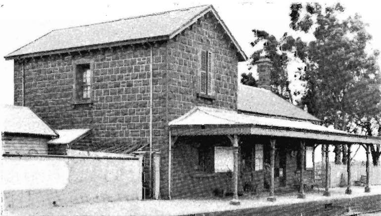
Lethbridge, a typical railway station building on the Geelong-Ballararat line.
