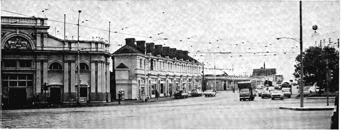
This could have been the site of Melbourne's major rail terminal if plans of 1859 had been carried out.
