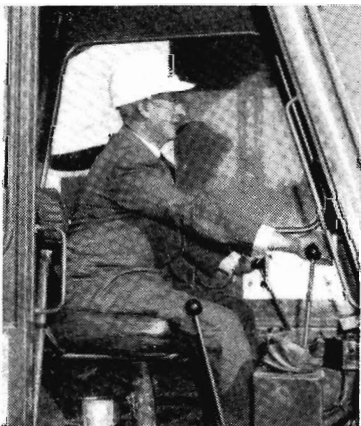
The Minister of Transport, The Hon. Vernon F. Wilcox, M.P., transports the first sod to a waiting truck.
