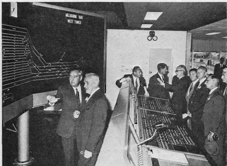
In the West Tower, the modern signalling panel held the attention of guests, who were given a tour of the new facilities before the formalities started.
