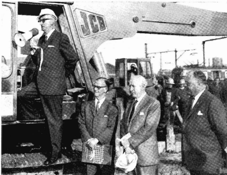
From the step of an excavating machine, MURLA Chairman, Mr. R. B. Roscoe, addresses the gathering at the ceremony to mark the start of the first ramp for the Melbourne underground. Standing beside him are (left to right) MURLA member and SEC Commissioner, Mr. T. P. Scott, Minister of Transport Mr. Wilcox; and Melbourne's Lord Mayor, Councillor Best.
