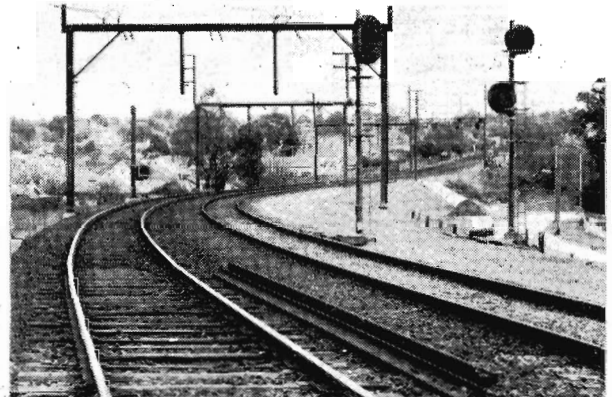
East Camberwell–Canterbury. Signals for the third line are already in position.
