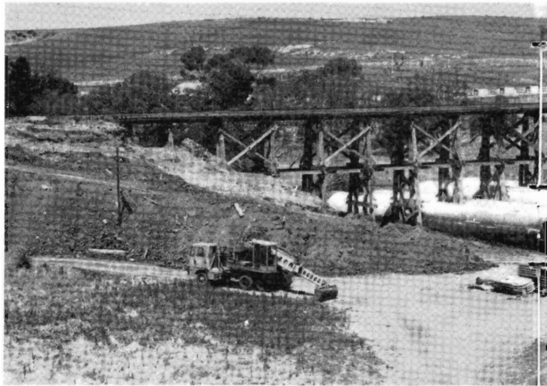
NOW YOU SEE IT ..... SOON YOU WON'T. By March, one of the two Marsh will have been replaced by Armco culverts. The increasing use of t
